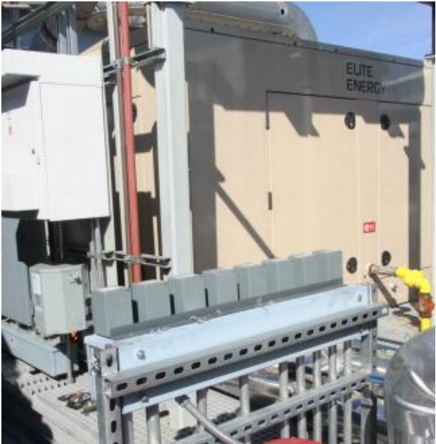
Cogenerator on the roof of the NAB. Photo from Prof Baglione’s faculty page.
